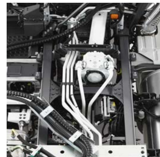
HYDRAULIC PUMP driven by the engine rear power take-off.
